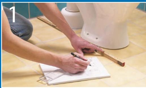
Measure the free floor area ie. excluding all floor standing units, to determine which size devimat is required.
