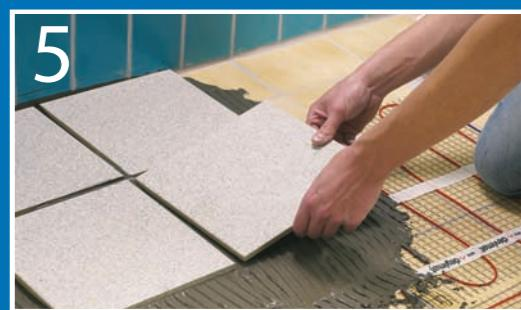
Cover with one layer of flexible tile adhesive/self levelling compound and allow to dry before tiling, or lay the tile adhesive and grout in one step. A flexible tile adhesive and grout should always be used.
