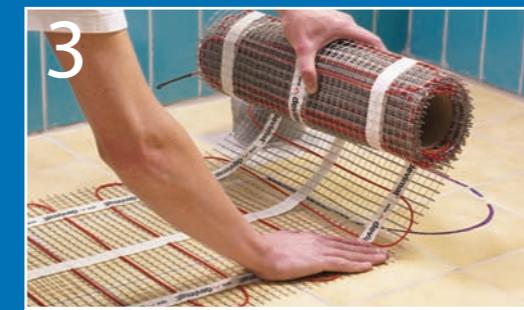
Before laying the devimat, the existing floor should be clean and dry, primed if necessary. Once the mat has been tested, it is then rolled out and laid onto the floor.
