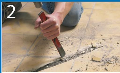
Cut a groove into the floor and wall 10mm deep and wide for the floor sensor and tube. The tube allows for easy removal of the floor sensor if required.
