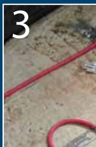
A piece of flexible tubing is used to connect the sensor led back to the thermostat.
