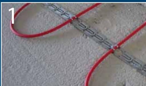
The devifast metal fixing strip is used to secure the heating cables.
