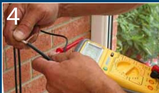
The heating cable and floor sensor are tested prior to screeding.
